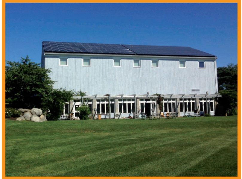
62.2kW Solar Plant Creates a Net Zero Campus
